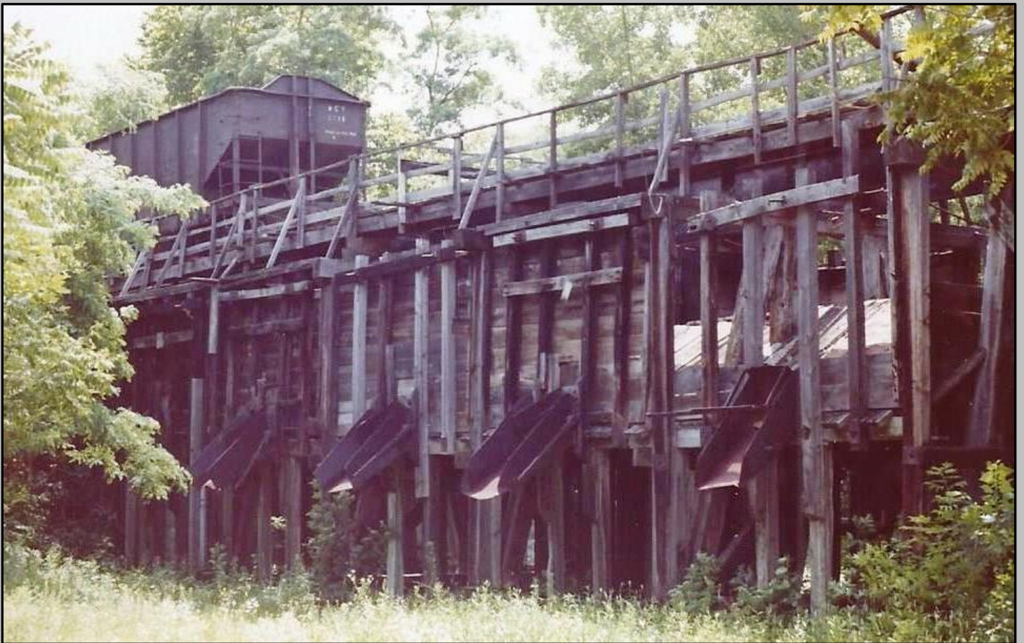
Above: The West Hill Coal Company was located just west of downtown Akron at Silver Street. The interesting wood trestle was still in service as late as 1980, though likely was used for limestone. At least three other coal dealers were located at or near Silver and North Streets in West Akron. Bob Lucas
