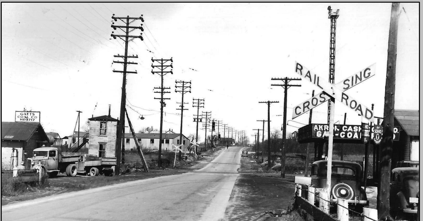
Above: Two retail coal dealers appear in this ca 1930's view at the far east end of Brittain yard. The dangerous grade level crossing of Darrow Road led to construction of a new Route 91 bridge over the AC&Y. AC&Y HS Archive
